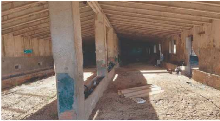
Vista interior nau 3
